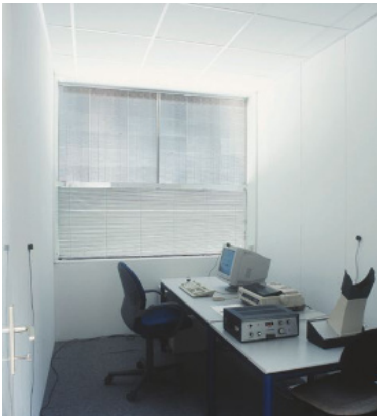
Fig. 7 Office with reflecting lamella system (no glare but daylight inside the room).
